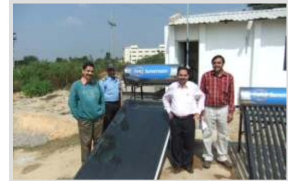
» Installation of solar panels at JAIN University
